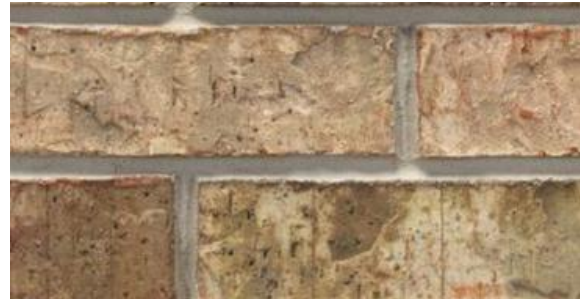
EXTERIOR BRICK: Acme Kennewick
